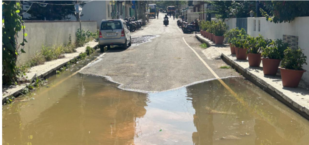
Sewage cesspool caused by the blocked drainage
