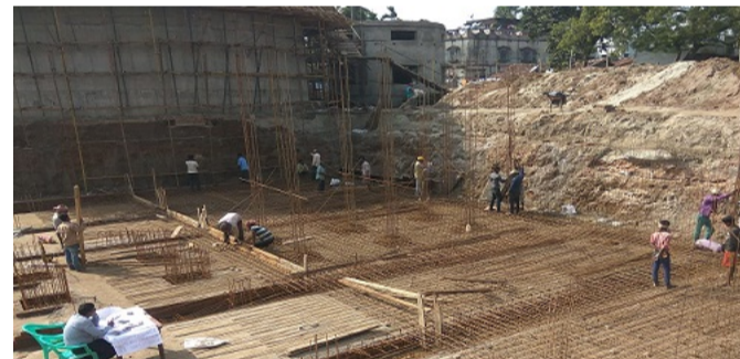
Ongoing construction at Howrah
